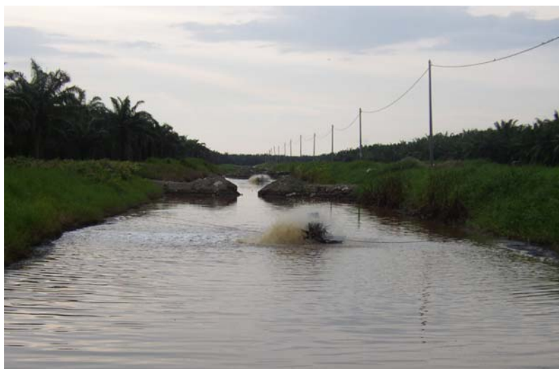
Figure 14.2: Pond for aerobic treatment of palm oil refinery effluent (Picture taken in United Plantation Berhad 2006).
